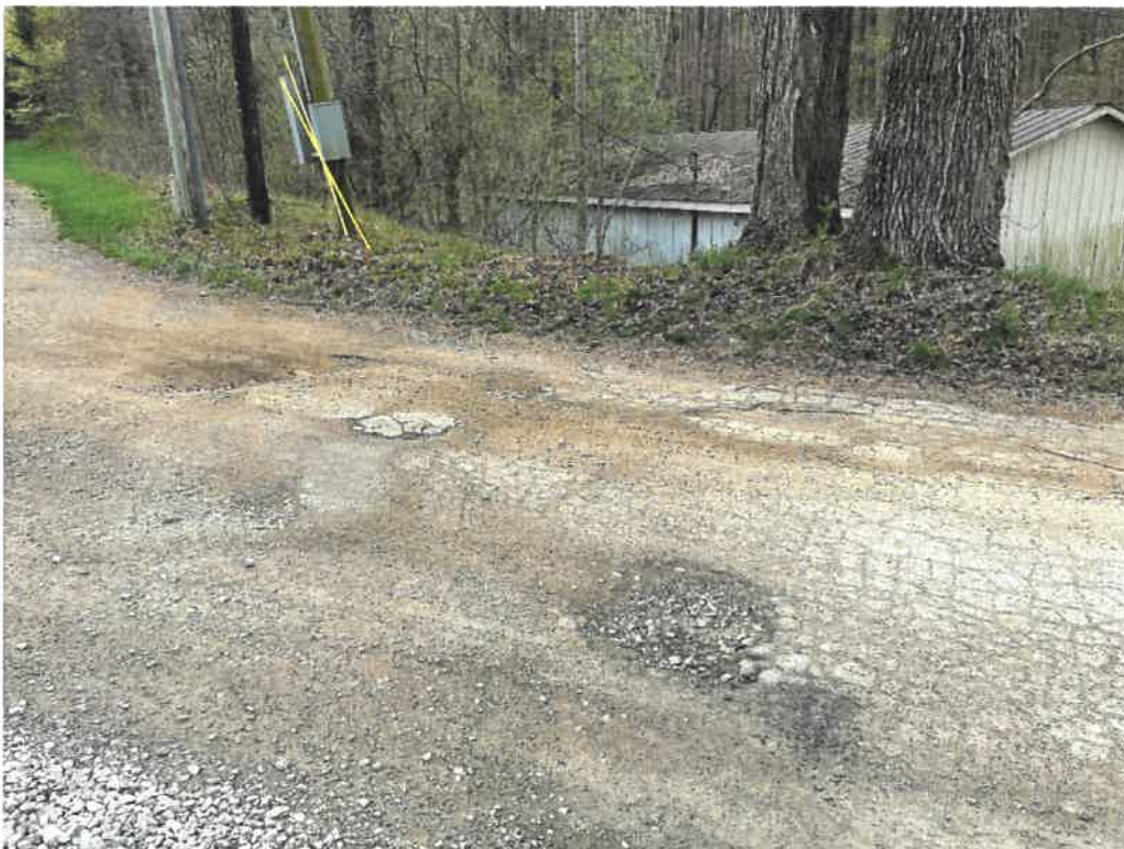
Tunnel Road potholes and alligator effect of failing asphalt. LLCD maintenance shed visible in background.
